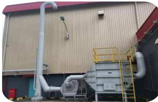
Picture 1. Activated Carbon Filter Unit for filtering the air from area of oil draining, dismantling and decontamination
